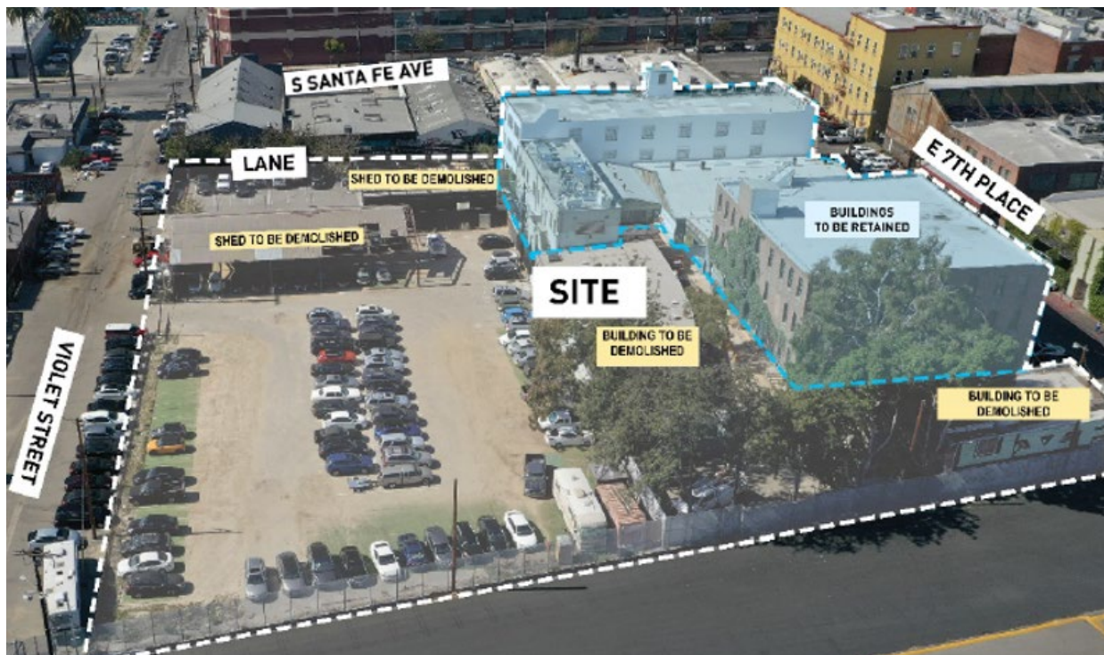
Aerial View of Existing Development
