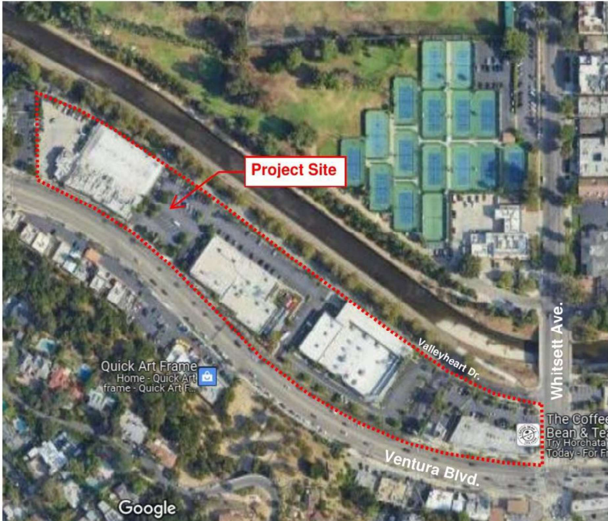
Figure 2 – Aerial Photograph of Existing Site Condition
