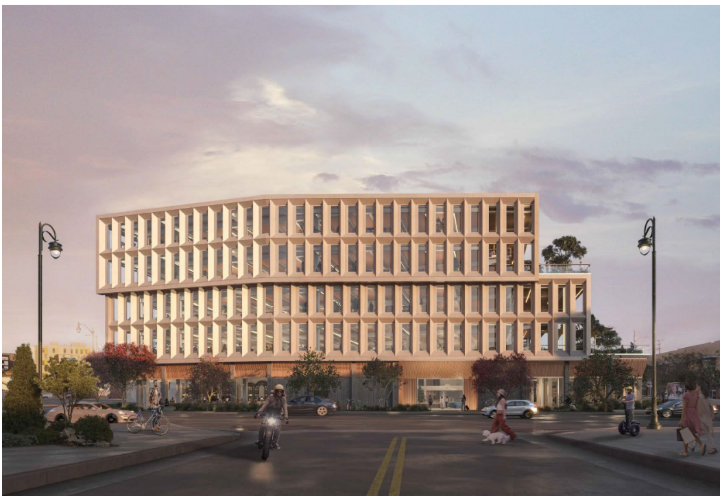
View of the West Façade from Alameda Street
