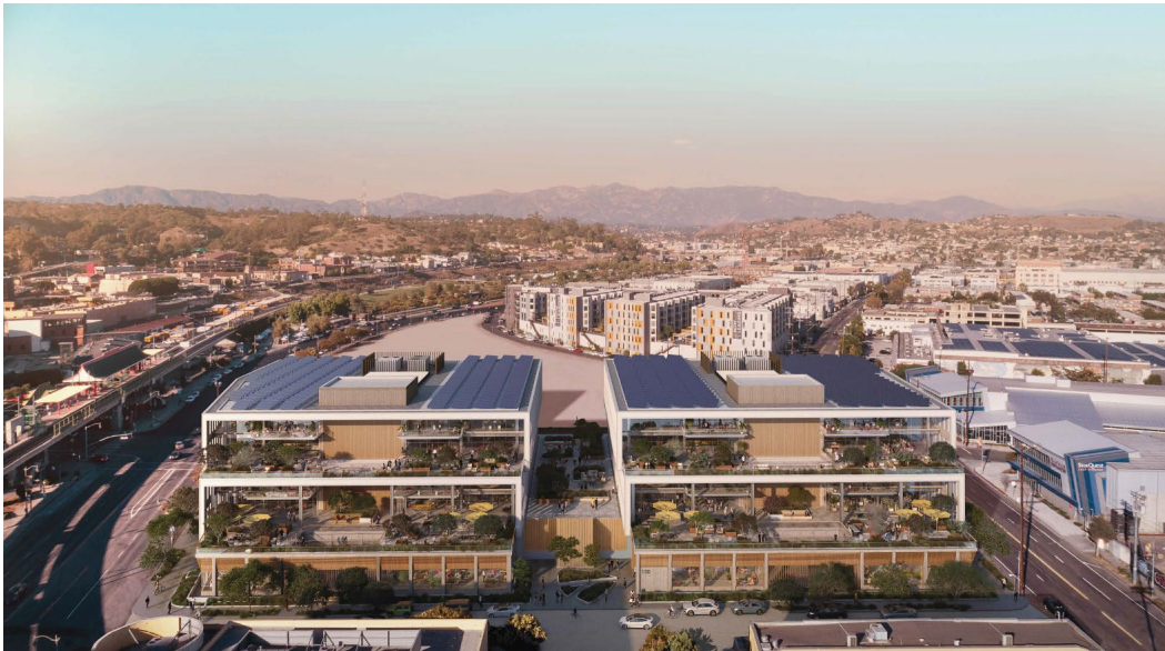
View of the Project from Bruno Street
