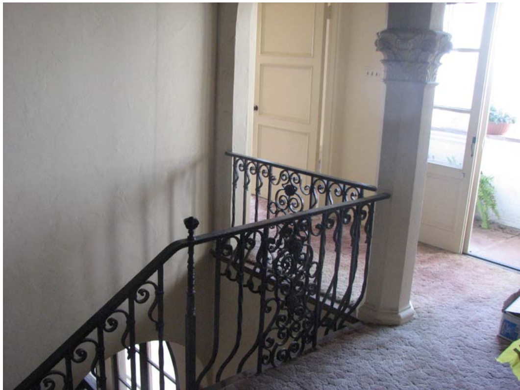
Victor Rossetti Residence, top of main stairs, 2188 Ponet Drive, June 14, 2007 (Charles J. Fisher photo)
