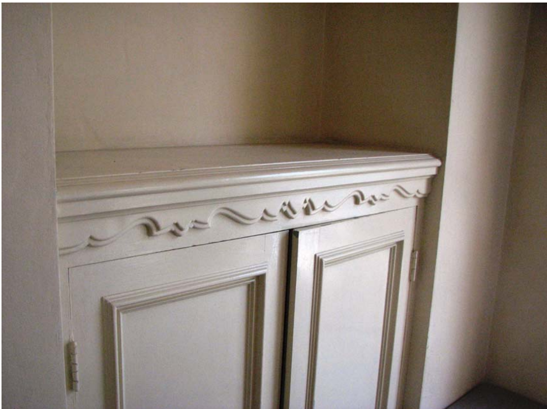
Victor Rossetti Residence, cabinetry, 2188 Ponet Drive, June 14, 2007 (Charles J. Fisher photo)
