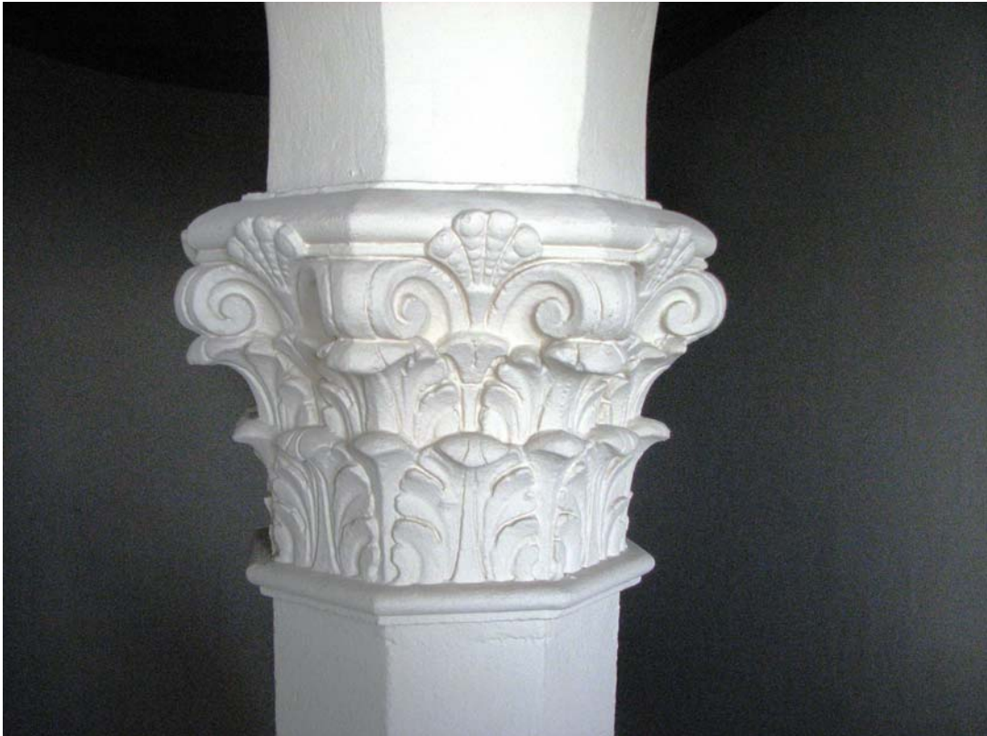
Victor Rossetti Residence, staircase column, 2188 Ponet Drive, June 14, 2007 (Charles J. Fisher photo)
