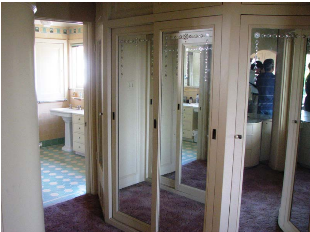
Victor Rossetti Residence, closets and bathroom, 2188 Ponet Drive, June 14, 2007 (Charles J. Fisher photo)
