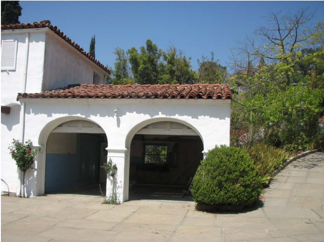
Victor Rossetti Residence, garage, 2188 Ponet Drive, June 14, 2007 (Charles J. Fisher photo)
