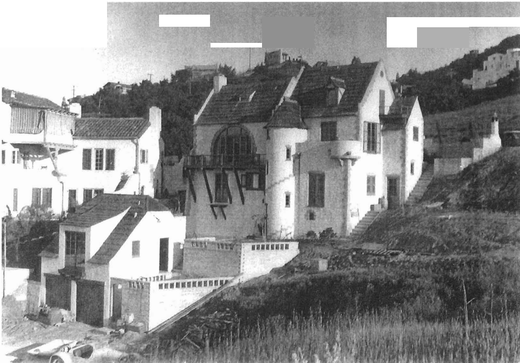
Exterior of residence nearly completed: Viewed to the southeast. Photo source: Estate of R. E. Hill ~ Date: 1927 ~ Photographer: R. E. Hill.
