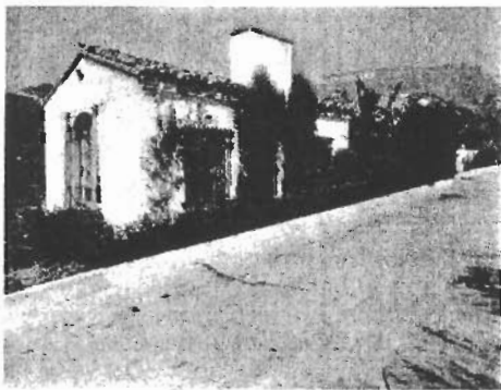
An original house after construction
