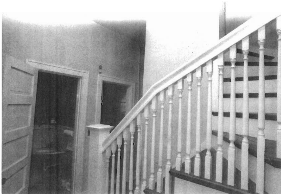
Rear service stairs with distinctive graduated balusters.
