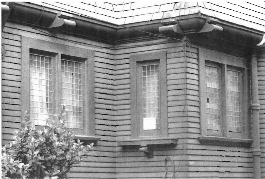
Southwest corner of residence with multi-pane leaded windows, viewed to northeast.
