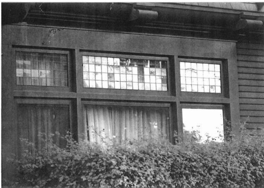
West façade library triptych windows with multi-pane leaded glass fixed transoms over single lights, viewed to east.
