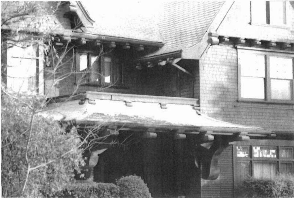
Projecting entry porch roof and second story recessed porch, viewed to southeast. Note decorative rafter tails and brackets.
