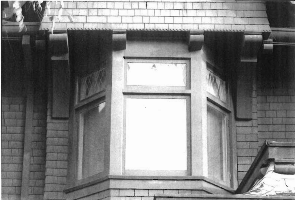
West façade second story slant bay window of master bedroom; fixed transoms with multiple leaded diamond lights over single lights, viewed to east. Note decorative shingle finish course, above.
