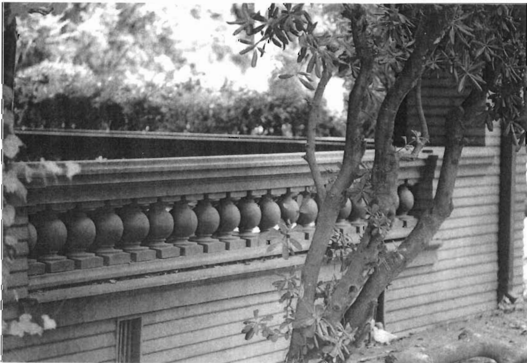
Detail: West façade porch, north balustrade, viewed to southwest.
