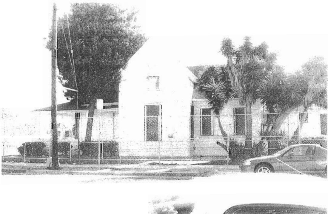
North elevation, viewed to south across Mont Clair Street.
