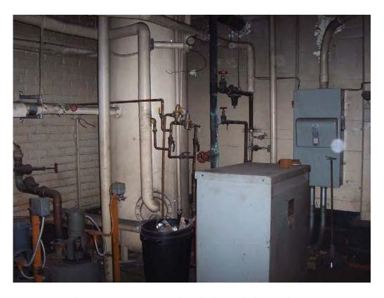
Photo 6. Hot Water Tank and Air-Cooled Transformer
