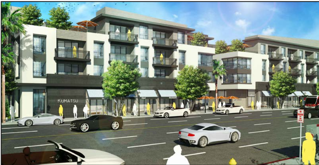
View of the South Mixed-Use Building from Reseda Boulevard
