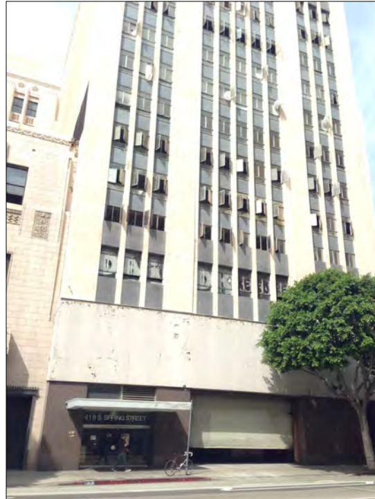
Figure 15: Property I, view northwest from Spring Street (McGee, 2017)
