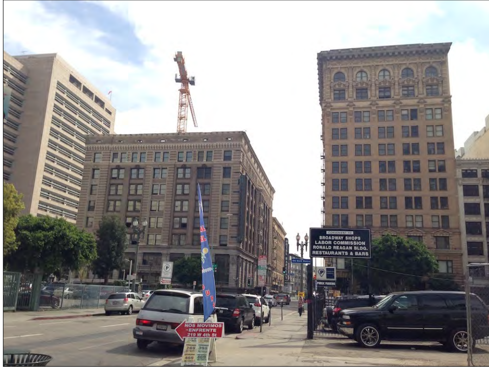
Figure 7: Banco Popular (Property E, left) and Continental Building (Property F, right), note subject property at right of photo, view northeast from 4th Street (McGee, 2017)
