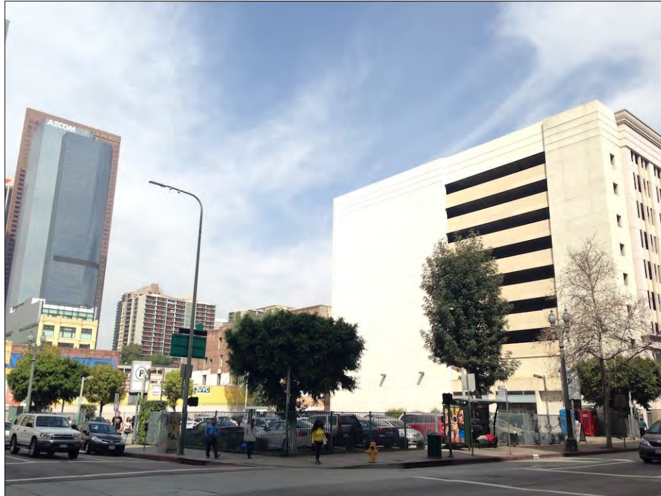
Figure 1: Subject property (Property A), view northwest (McGee, 2017)
