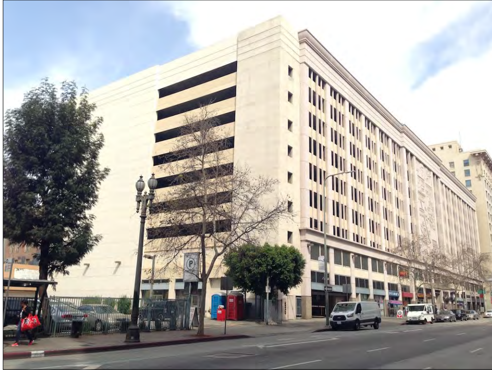
Figure 3: Broadway Spring Center (Property B), view northwest from Spring Street (McGee, 2017)
