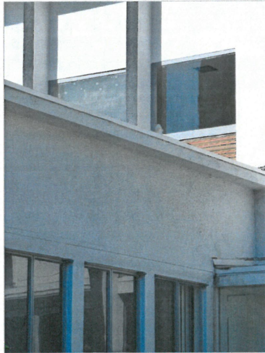
Figure 5 Detail, east elevation, showing tile wainscoting and replacement wood-frame windows at second story above one-story wing
